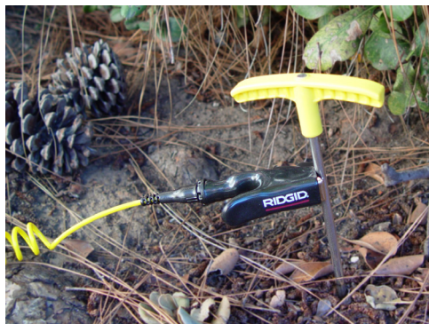
Figure 6 – Lead clip attached to the ground stake
