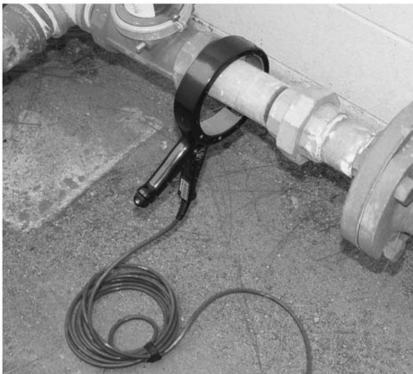
Figure 4 – Example: Attaching The Inductive Clamp
